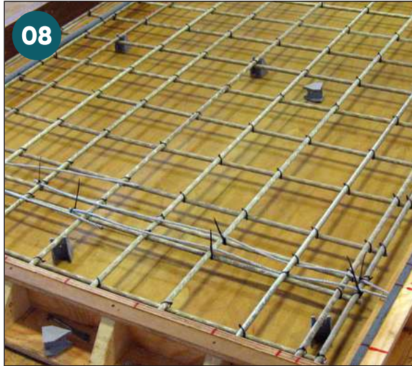
Civil Engineering Work
